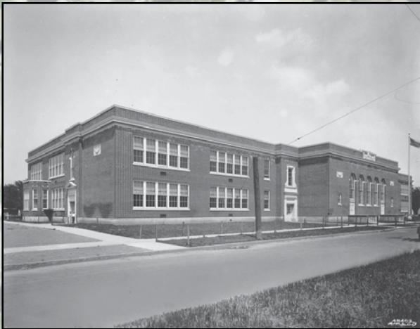
1924 photograph of Abernethy School, looking north
