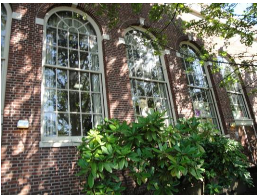
East elevation auditorium
