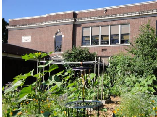
West elevation and garden
