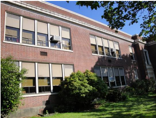
East elevation entry
