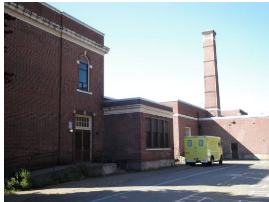
Gymnasium west (rear) elevation
